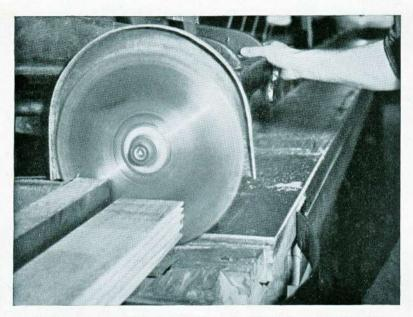
A single saw cut-off trimmer showing a bundle of clears going through
