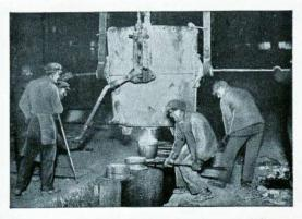
Pouring Electric Furnace Steel from one of the 6-ton ladles
